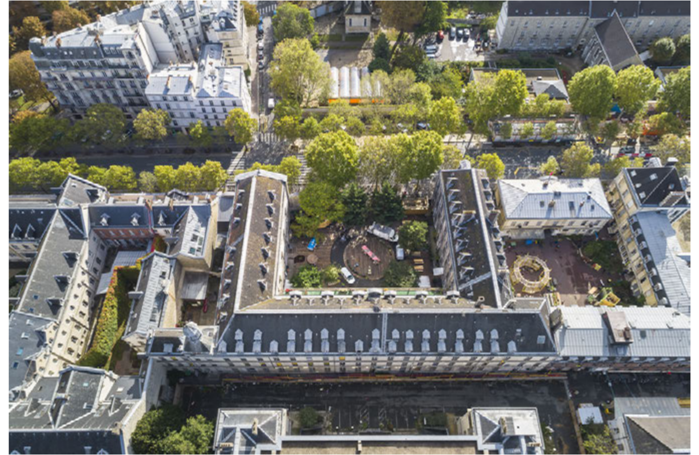
Overhead view of the Robin and Oratory buildings, showcasing the preserved historical façade (Source: Sergio Grazia from Ville de Paris website )
