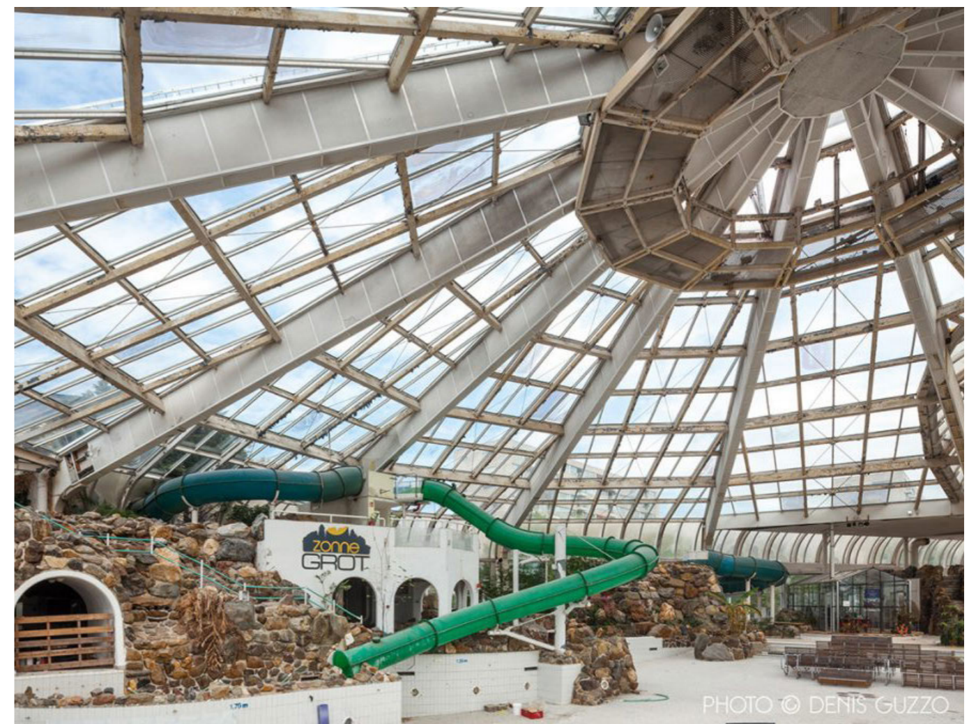
Before and after image of the tropical swimming pool dome (Source: Denis Guzzo, Stadsarchief Rotterdam and SuperUse Studios )
