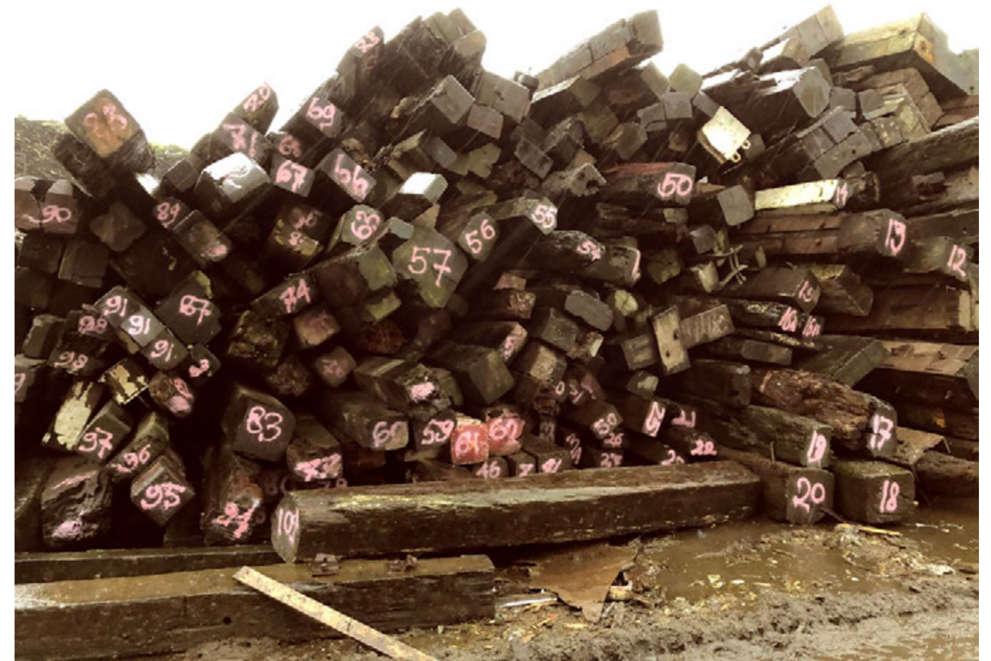
Wooden fender poles were specifically identified and measured so that the linear programming model could optimise their shape and layout on the final structure (Source: Boris Zeisser)
