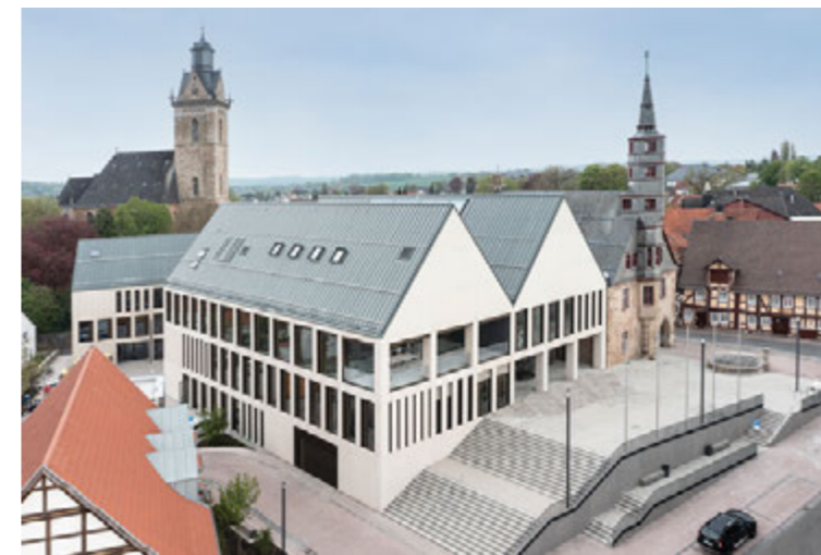
The building extension from the 70s was replaced (Source: Anja Rosen, AGN )
