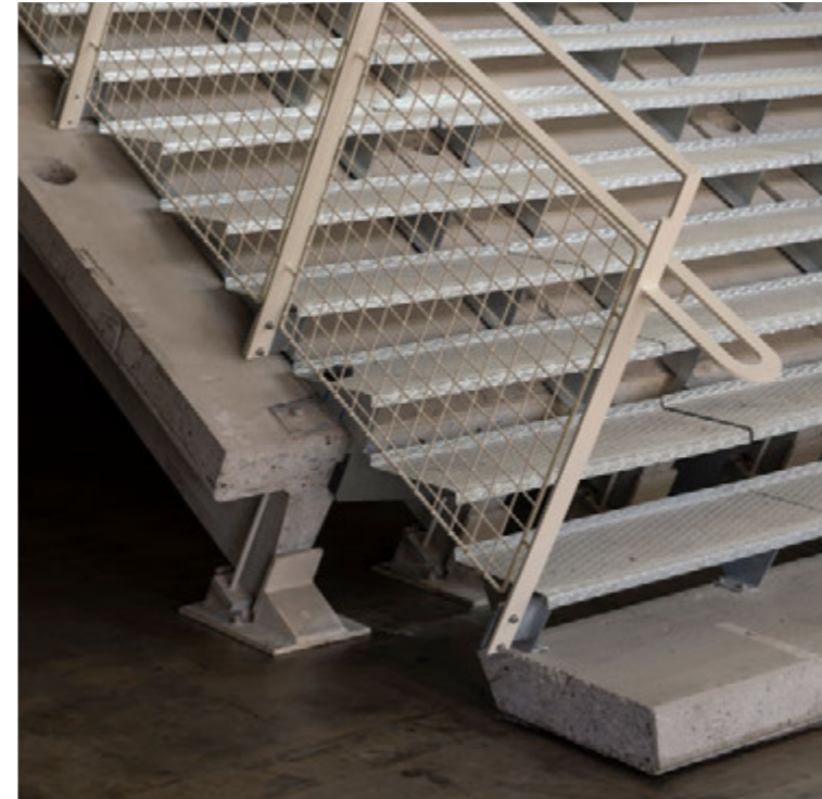
Images showing the concrete slabs from the original floors being cut and tilted to fit new stairways (Source: Hampus Berndtson)
